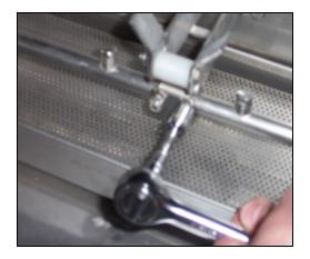
Removing the lower rinse arm support bracket
